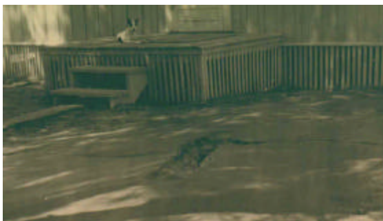
Fig.3: 1950 Sand boil deposit near house about 1.5 km northwest of WLA site
